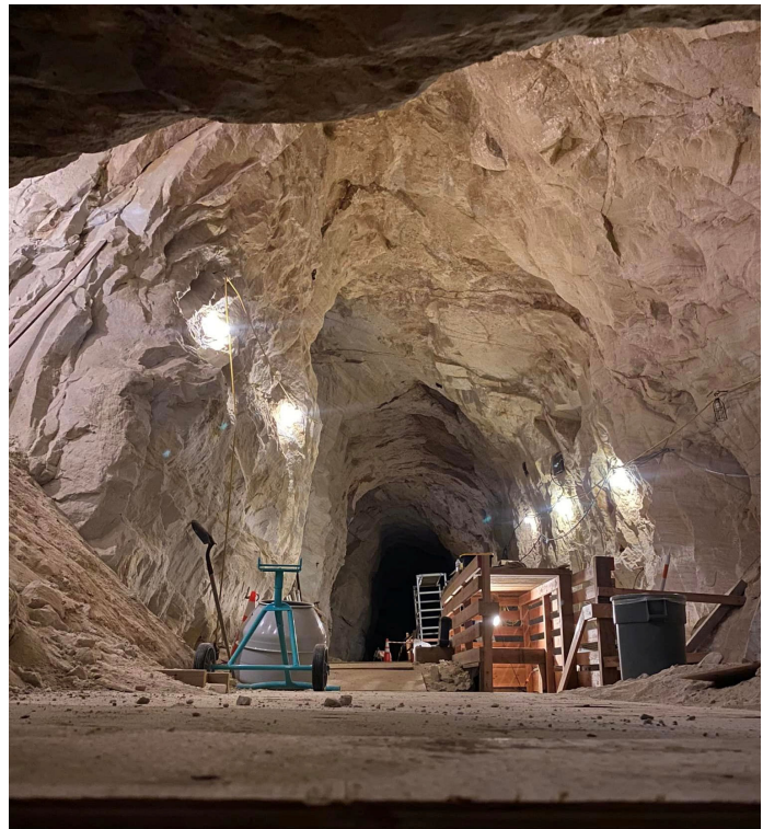
MINE REPAIRS ARE ALWAYS ON GOING
