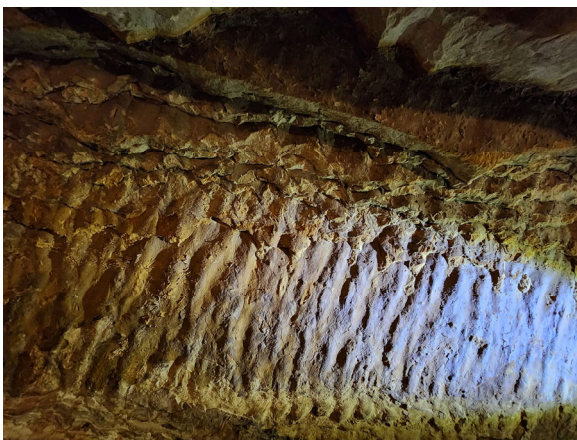
RIPPLE MARKS IN SANDSTONE ON ROOF OF TUNNEL
